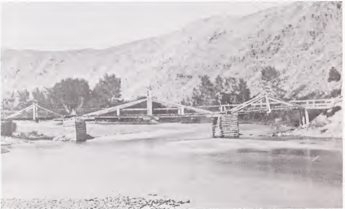
The original Browne's Bridge over the Big Hole River. It was the last operating toll bridge in Montana. The King Post trusses and rock crib piers were typical of early bridge structures in the state (Montana Historical Society).
